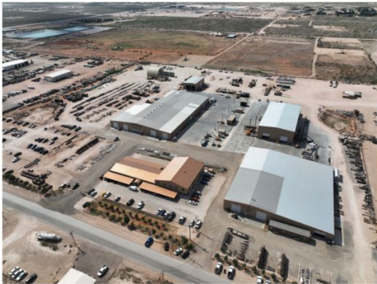
Fabrication Facility – Midland TX
